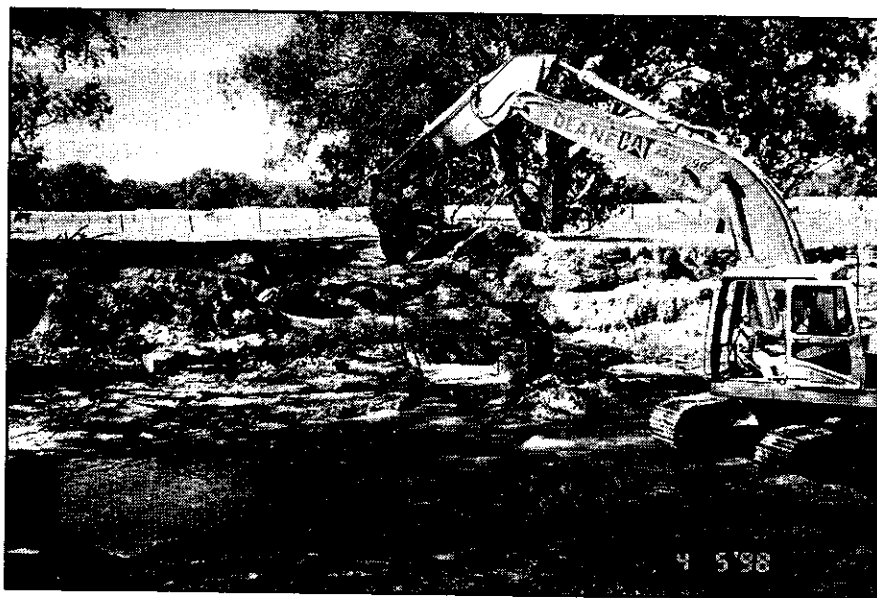
During installation: A trench was excavated and the logs buried to half their diameter. The root balls were buried into the bank. Photo courtesy of Peter Davies.
